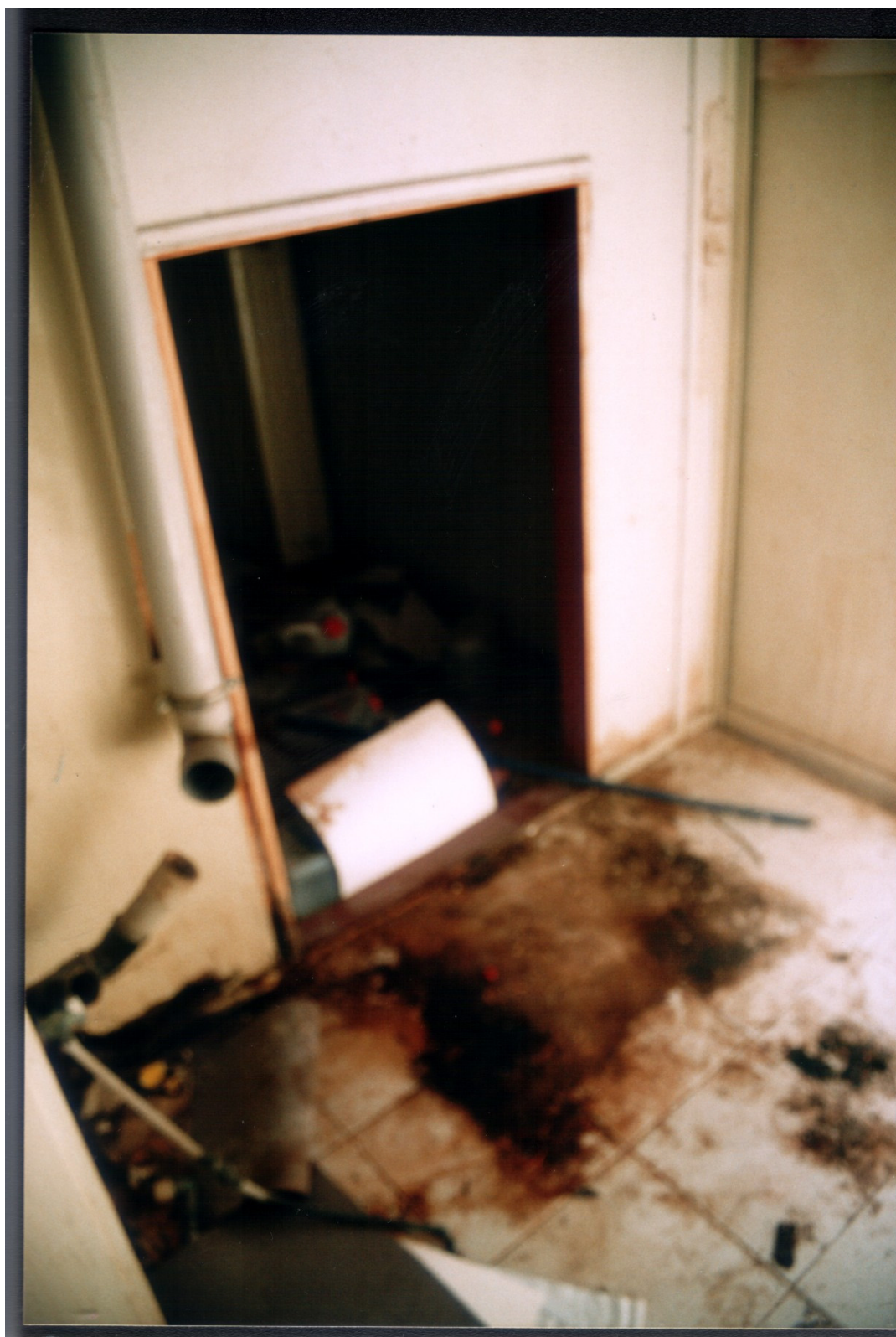
Figure 1 Stains from processing chemicals (photo of development room).
